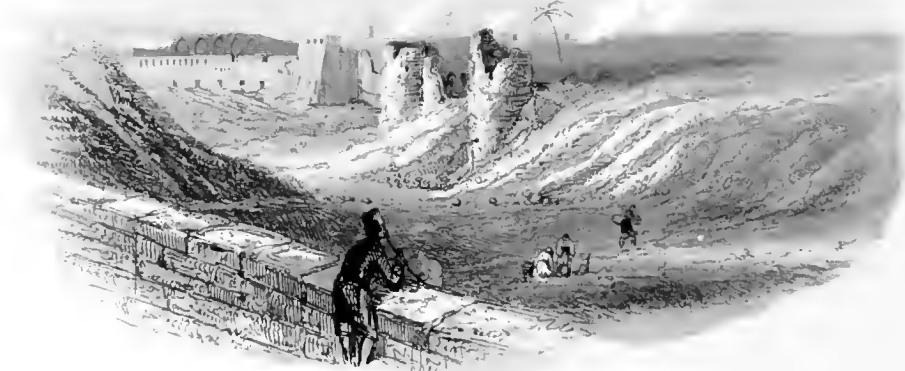
Inner Breach looking South
